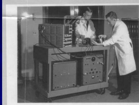
1951—Wild and Reid conduct a real-time B-mode sector scan of Wild's wrist using the prototype B-mode equipment built out of spare parts in Wild's basement. This equipment was later used to detect cancer in patients.
